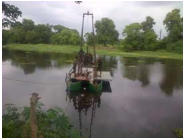
Boring work at Puzhakkal Thodu
