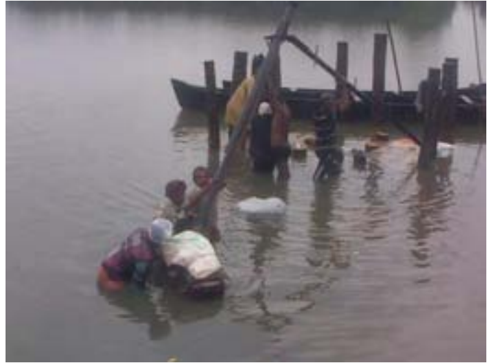
DCPT work in progress at Azheekkal
