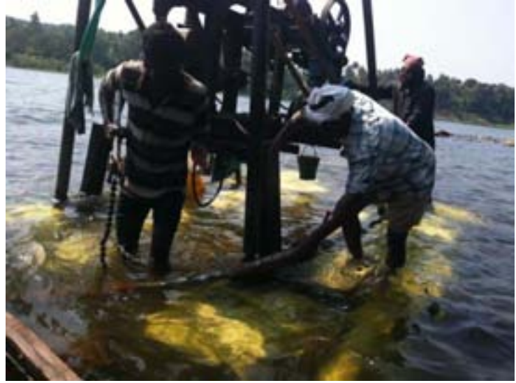
Boring work at Bhoothathankettu
