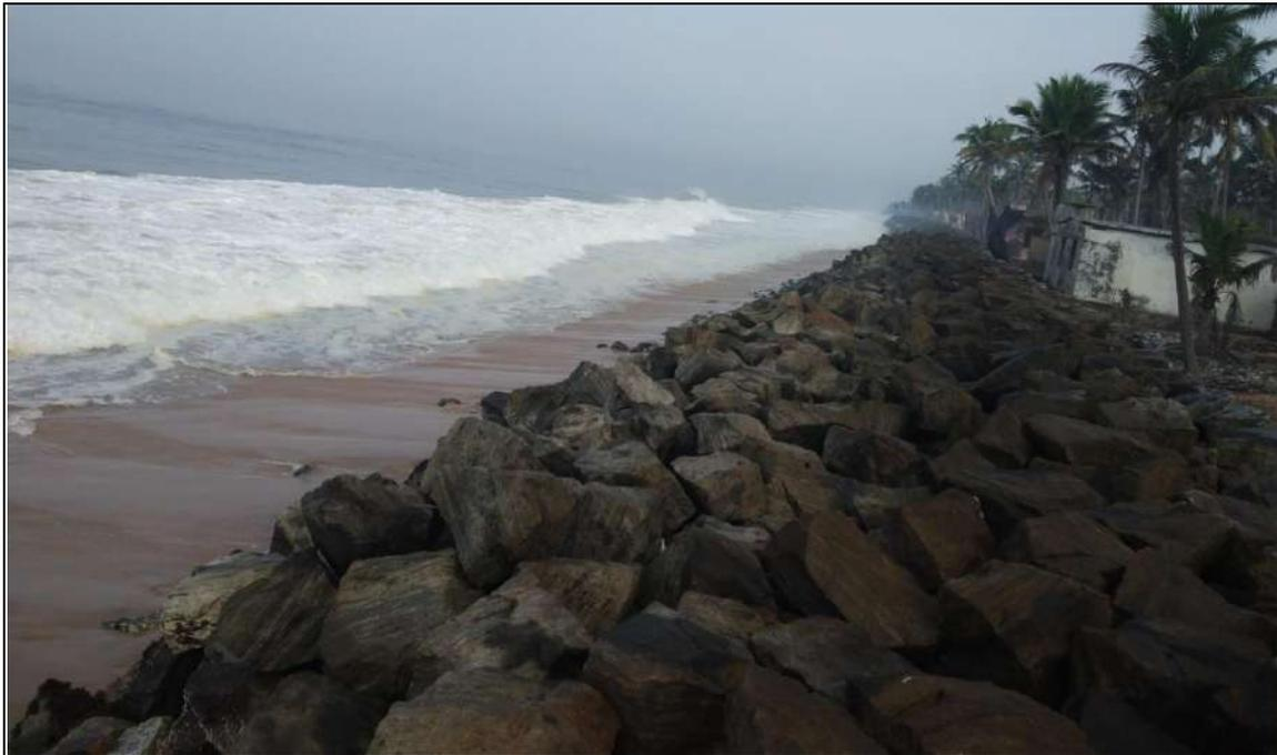
Although heavy flood occurred during the month of August of this year, no heavy damages reported in the coastal region. At the time of OCKHI, the entire region both sea wall and nearby houses were damaged severely. This portion is now under the construction of 15 numbers of groins to avoid further damages. The damaged houses are still in the condition as such.
