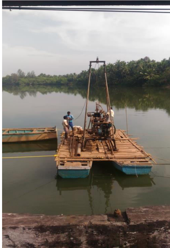
Boring work in river
