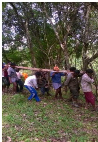
Shifting of Boring plant
