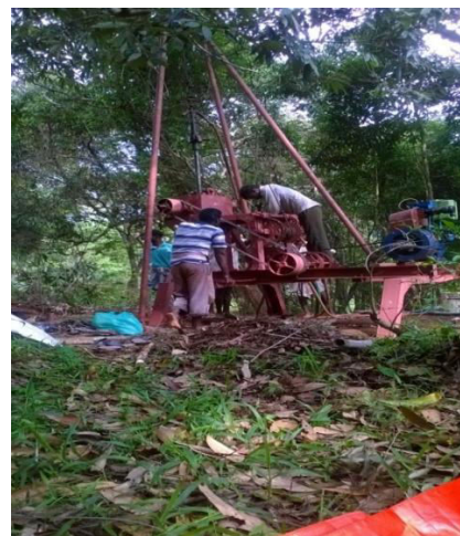
Setting of boring plant
