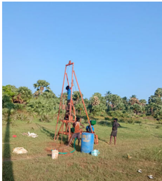
Soil Investigation at Kunnampidari Eri
