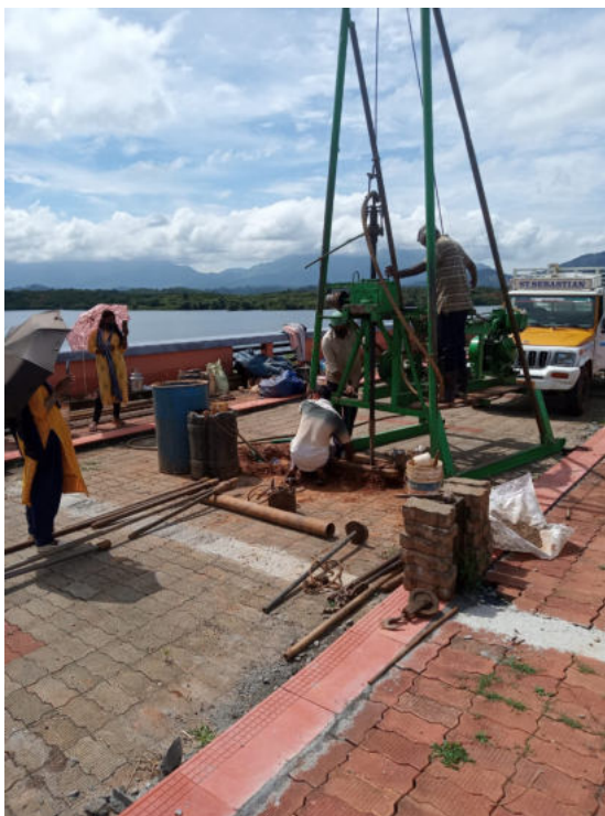
Supervision of the soil Investigation of Karapuzha Dam
