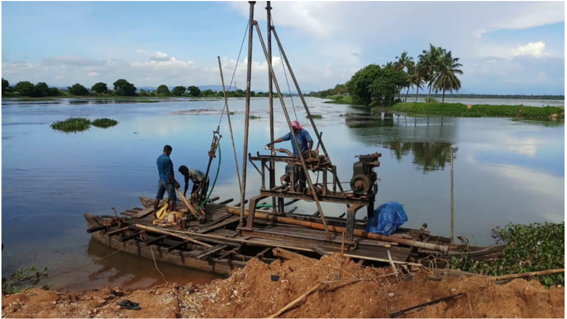
Soil Investigation at Enamakkal Regulator, Thrissur District
