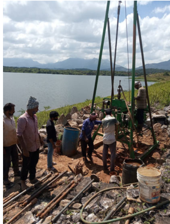
Supervision of the soil Investigation of Karapuzha Dam
