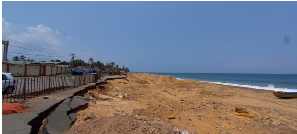
Maintenance work going on at Sangumukham
