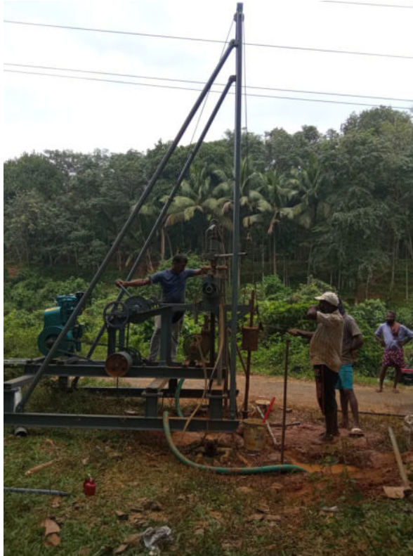
Soil investigation at Ch.17 km at KIP main canal, Pathanapuram, Kollam District
