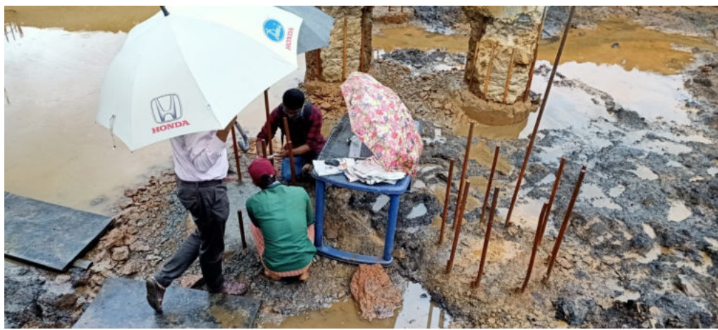
Fig 2. Pile Integrity Testing at Karichal Kadavu, Kunnamkulam
