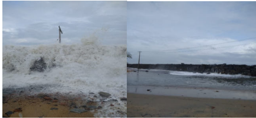
Fig 2: Overtopping and Under scouring witnessed at the Edavanakkad region during monsoon
