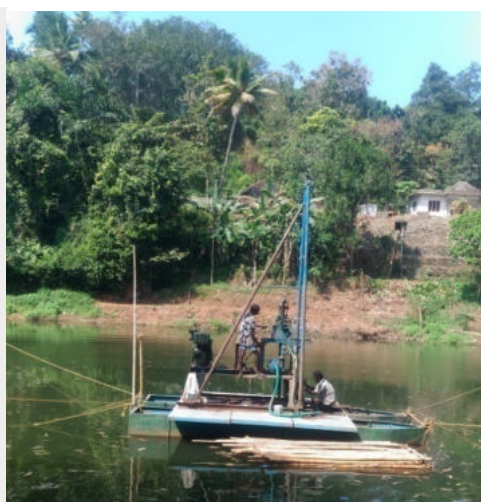
Diesel Boring Plant
