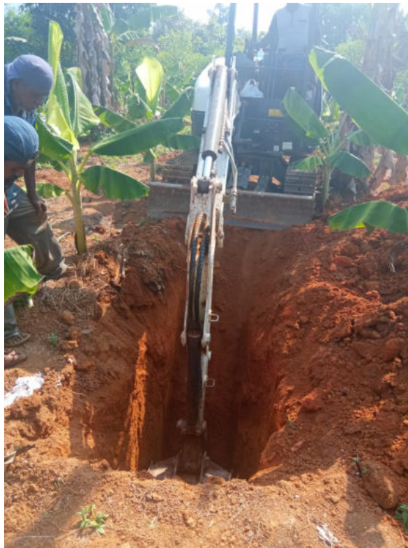
Soil Investigation Works - Development of Fish Seed Hatchery at Bhoothathankettu
