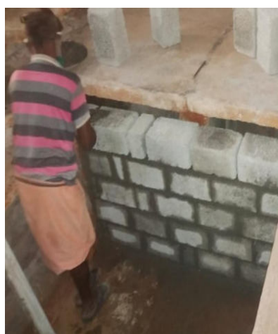
Construction of Initial setup
