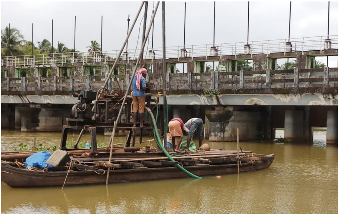
Soil Investigation at Idiyanchira Regulator, Thrissur District
