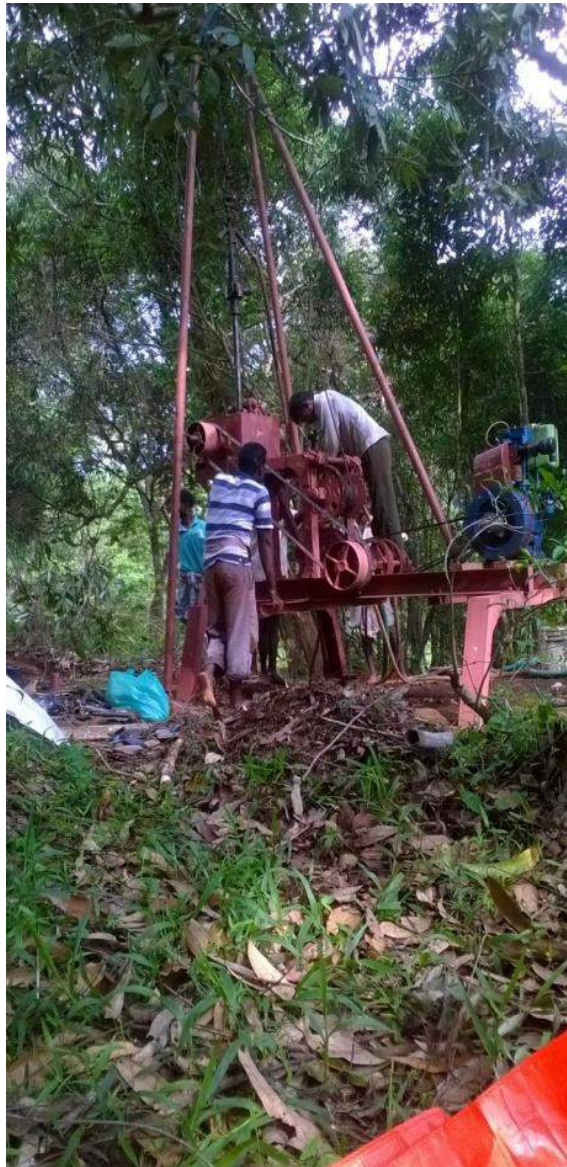
Setting of Boring plant at Mullaperiyar site
