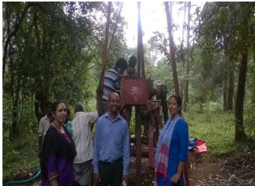
Ready to start work
