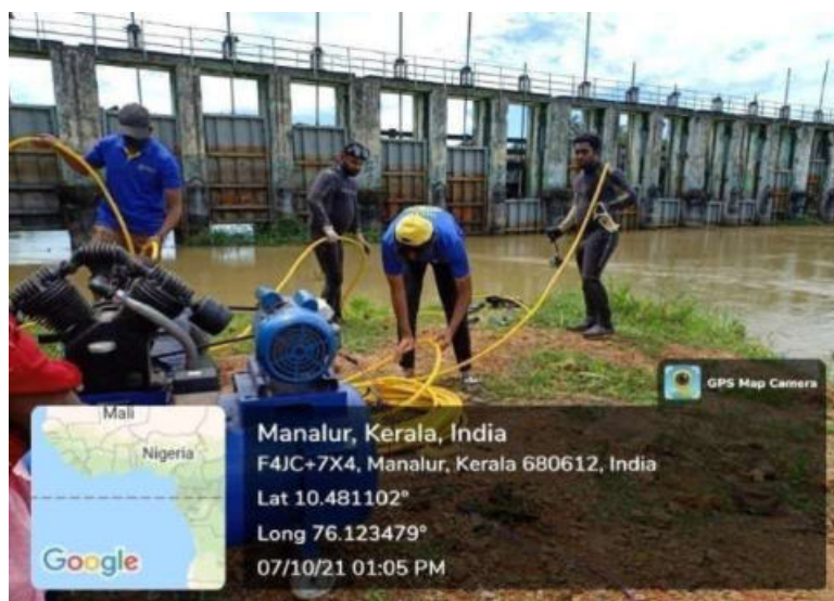
Preparation for underwater inspection at Upstream side
