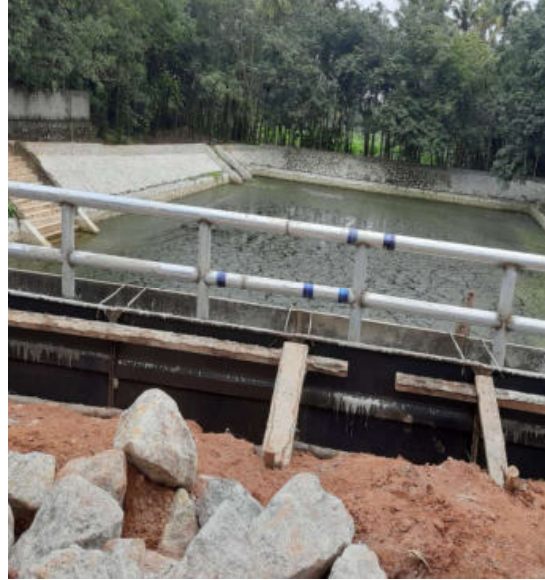
Renovation of Pond – M.I. section Chathannur
