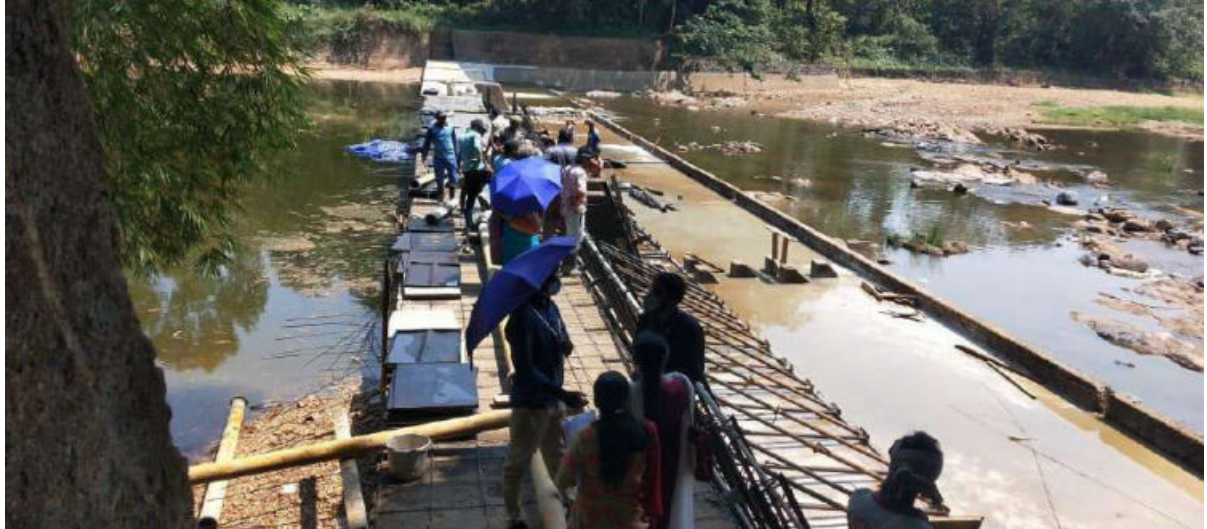
Lining work of Moonganicheckdam under Irrigation section Kanjirappally
