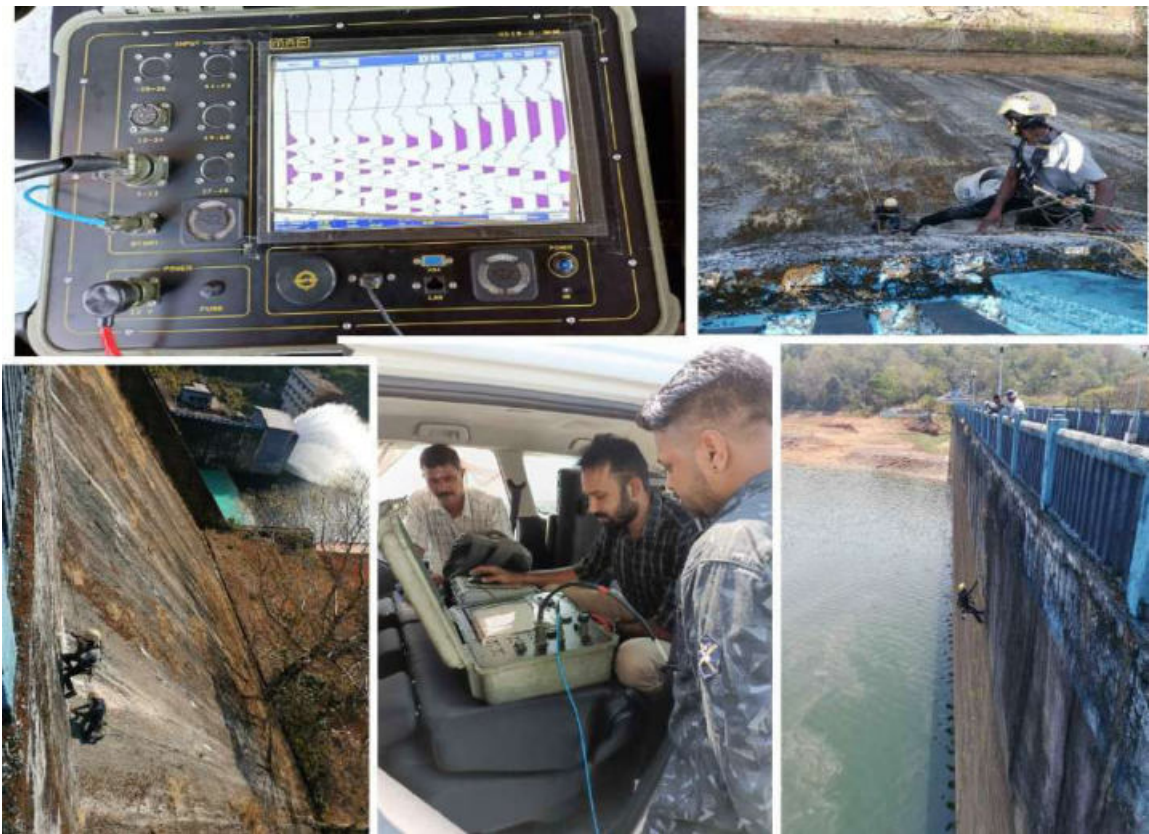
Fig 19. Seismic Tomography study at Chimoni Dam
