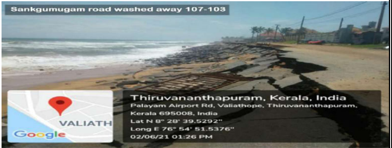
Sangumukham Beach Road-Before&After construction of RCC DiaphragmWall
