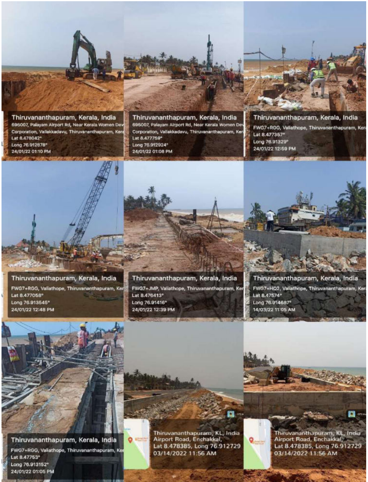
Construction of diaphragm wall going on photos at Sangumukham
