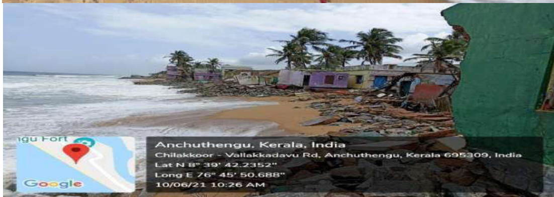
Damaged houses at Anjuthengu
