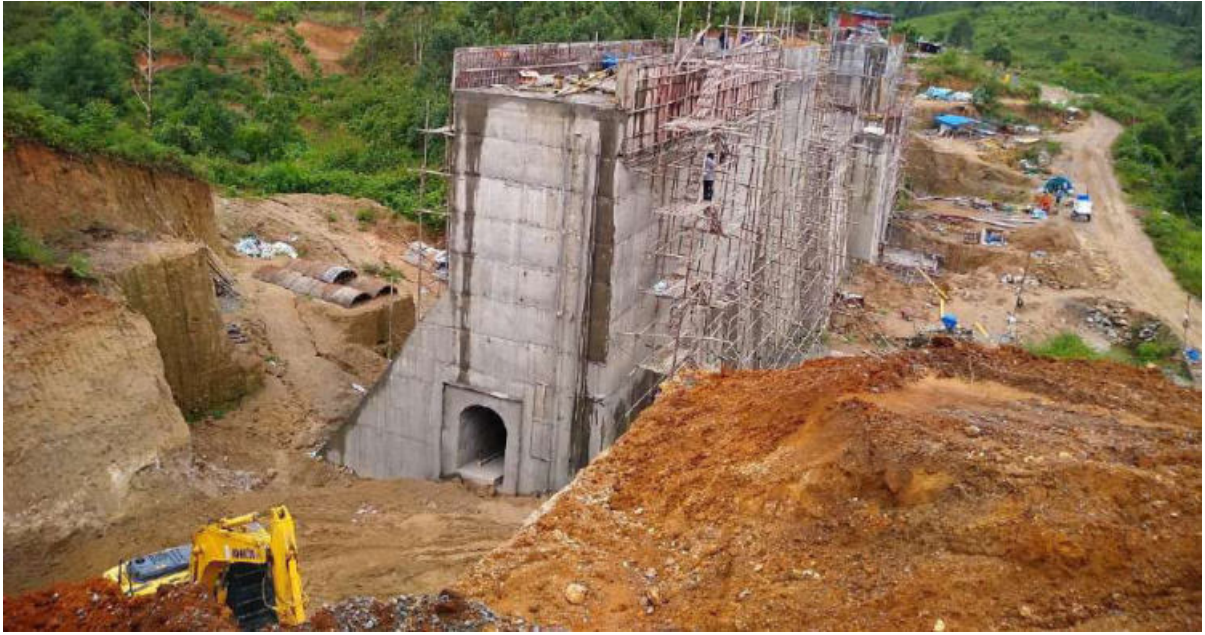
Construction of Pattissery dam
