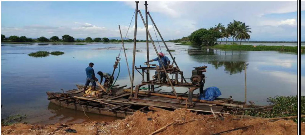
Fig 1. Boring Using Rotary Calyx Drilling Machine
