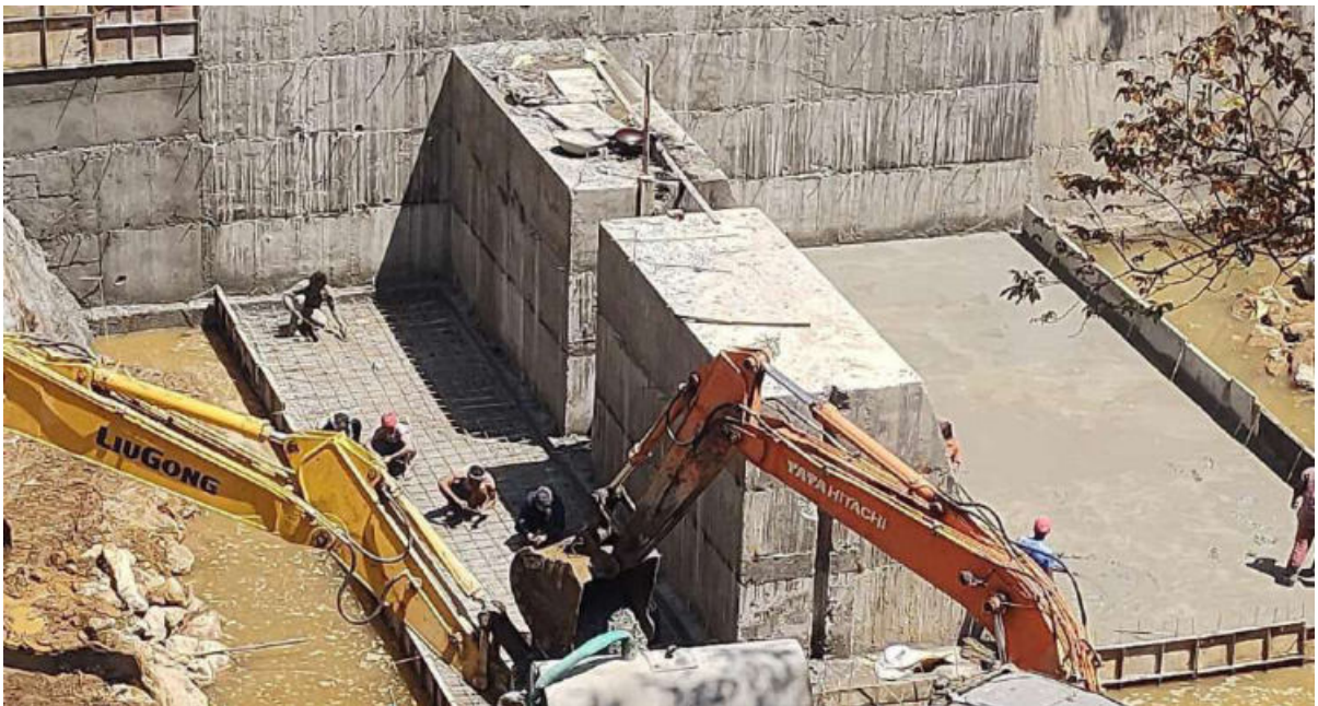
Construction of Pallivasal Checkdam
