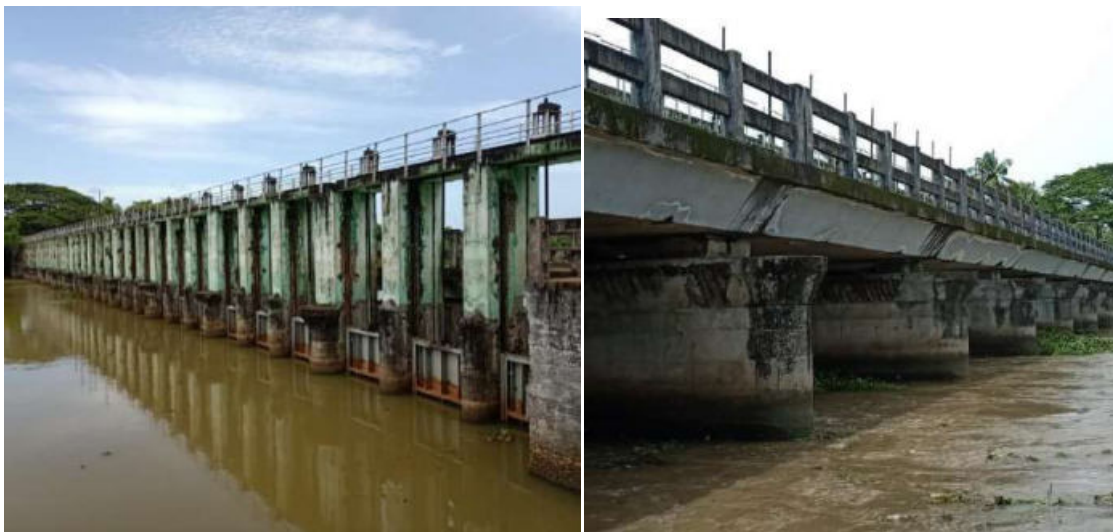
Upstream and downstream view of Structure
